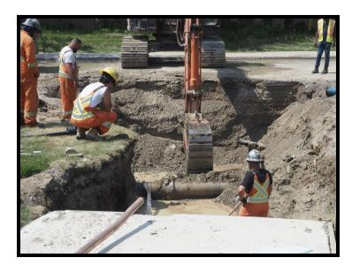
Meanwhile at the front of the Leslie Log House property, the City is digging a trench to replace the existing water mains. Our brand new sidewalk, which was installed only last summer has had two or three sections dug up at the edge of the front garden and the crew is busy trying to dig out the old pipe. Hopefully this will all be over and done with shortly!
