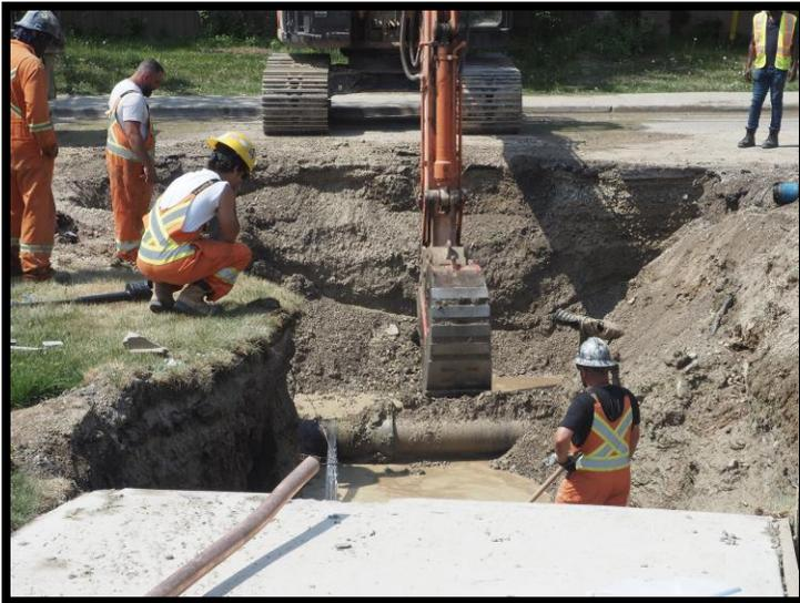
Meanwhile at the front of the Leslie Log House property, the City is digging a **trench** to replace the existing water mains. Our brand new sidewalk, which was installed only last summer has had two or three sections dug up at the edge of the front garden and the crew is busy trying to dig out the old pipe. Hopefully this will all be over and done with shortly!
